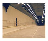
Tunnel Panels – The precast polymer concrete barrier is available in modified shapes for use as bench wall, corrosion and impact protection.
